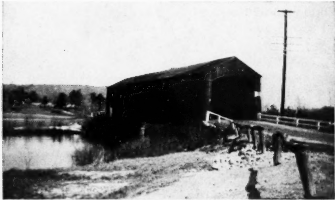
Covered Bridge in Partridgeville Section of Athol, Mass.
